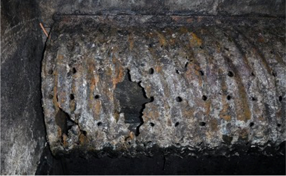
Figure 1- Corroded 72" wide corrugated steel trash screen.
