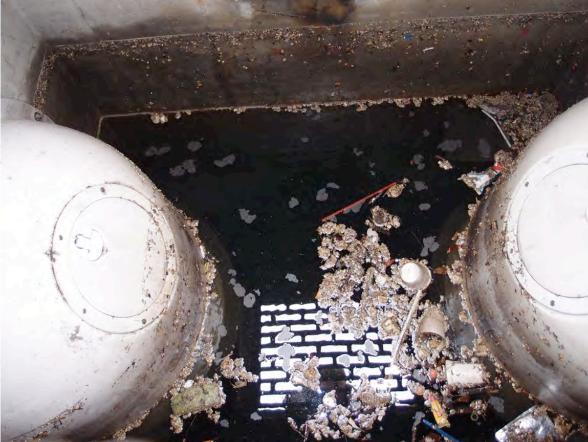
Figure 7, Near 3 rd Avenue S., and Ocean Boulevard. Shown is a pair of 30F SNOUTs covering 24” perforated pipe
