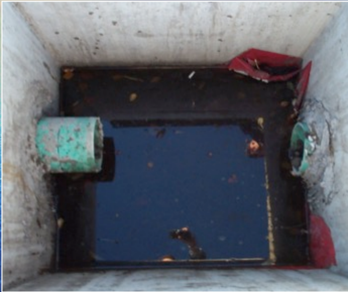
Inlet shown with no SNOUT that flows into structure with SNOUT. Water clear, no oil, little trash.
