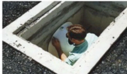
SNOUT is Trial Fitted over Pipe
