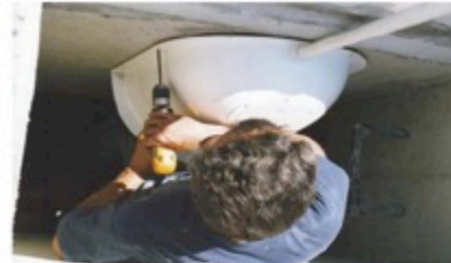
Holes Drilled for Anchor Shields
