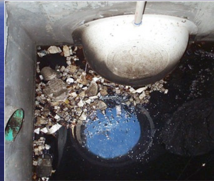
Structure with SNOUT stopping trash, oil and debris from upstream.
