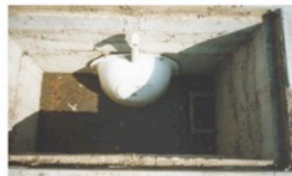
The SNOUT Trapping Floatable Oil and Debris
