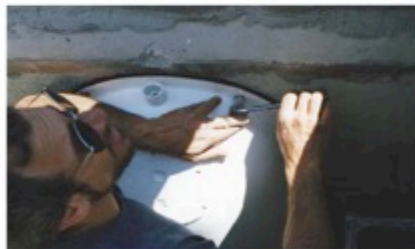
SNOUT is Bolted to Wall with Gasket on SNOUT Flange
