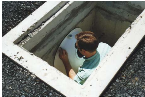
SNOUT is Trial Fitted over Pipe
