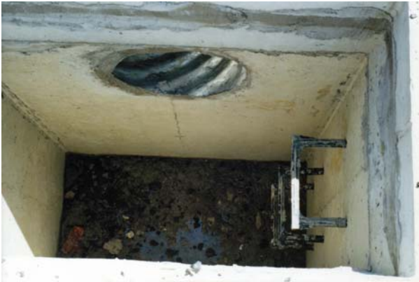
Empty Structure is Prepared
