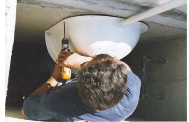
Holes Drilled for Anchor Shields
